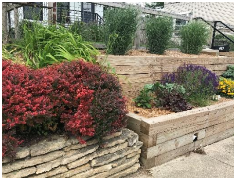
Taller tiered walls in a variety of materials. Retaining walls over 4 ft. require stamped drawings and a building permit.
