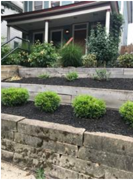
Taller tiered walls in a variety of materials. Retaining walls over 4 ft. require stamped drawings and a building permit.
