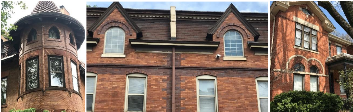
The brick is fired and has a hard surface – more impervious to the elements
