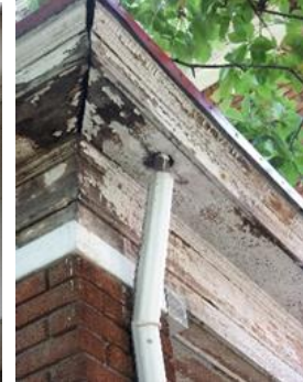
Separated Downspout
