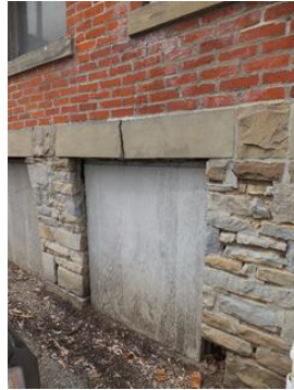
Cracked Lintel
